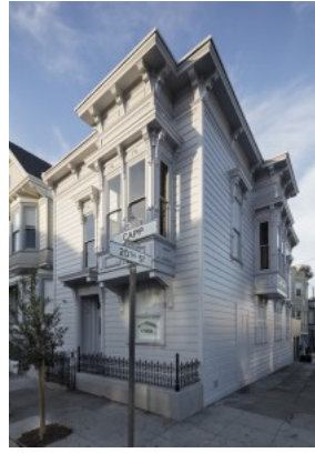
10 David Ireland, exterior view of House, 2015.
